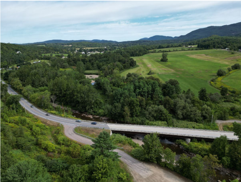
New Haven River and Route 116
