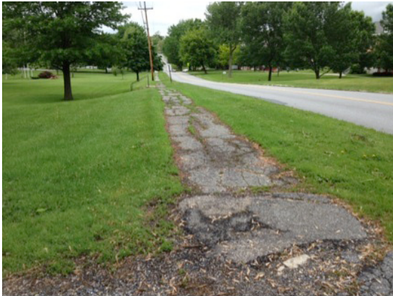
3. Asphalt roadside sidewalk in poor condition
