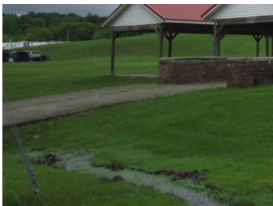
7. Roadside grass "swale" in poor condition
