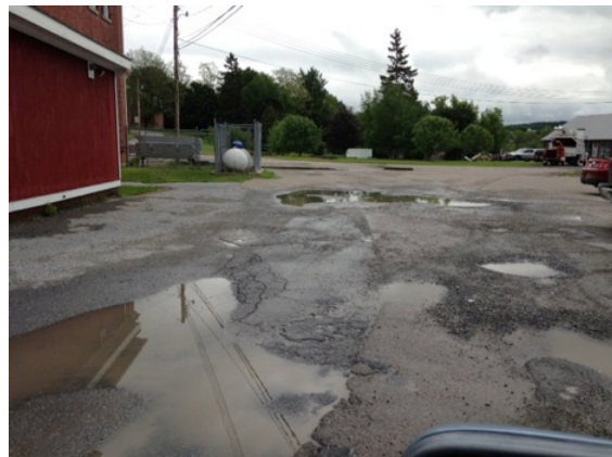
6. Pooling water on interior road network/parking area
