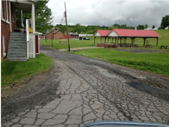
1. Asphalt and gravel interior road in poor condition
