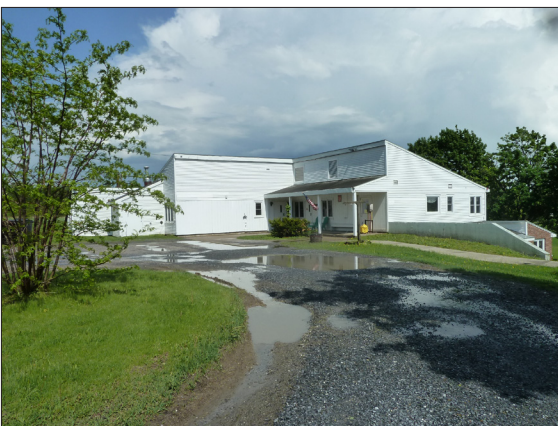
11. Ponding and erosion at a newer dormitory site
