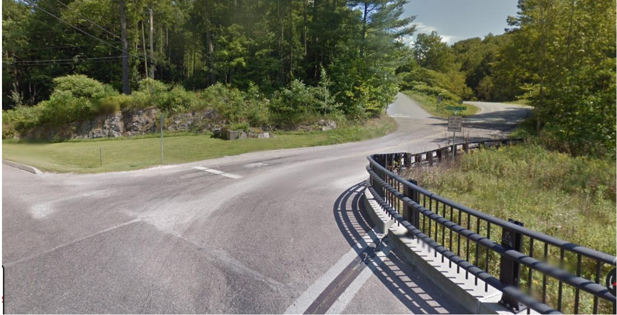
Briggs Hill descends at almost 10% grade and intersects Lincoln Road at an acute angle. Coming down or going up Briggs Hill is always a crap shoot. The Stop Sign is frequently run. This also makes the left hand turn on to Briggs Hill dangerous.
