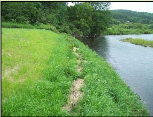
FES with Stone Fill, Floodplain Bench
