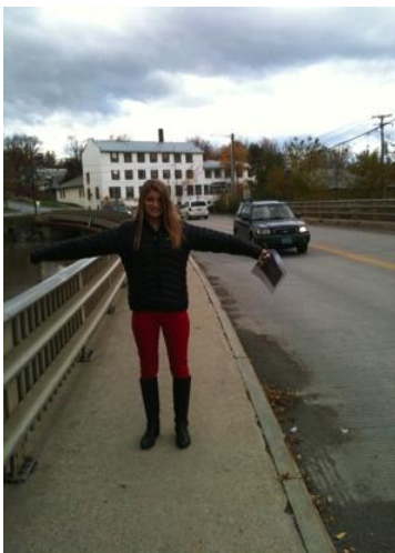
Figure 1.6: The 4.5 ft wide sidewalk on Otter Creek bridge
