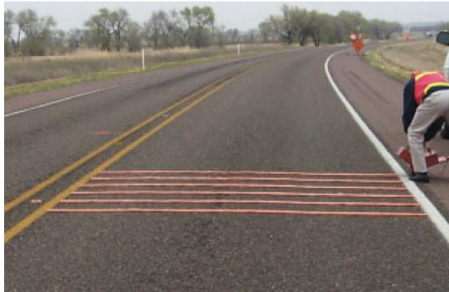
Figure 6.11: Rumble strips, an example of textured road surfaces
