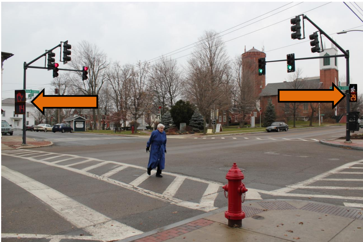
Figure 6.1: Addition of Pedestrian Signals at the Junction of Main Street/22A and Green Street
