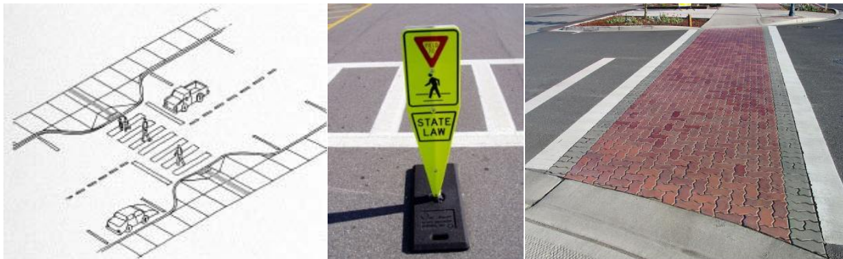
Figure 6.3: Crosswalk "bump-outs," in-street crosswalk signage, and cobbled texture
