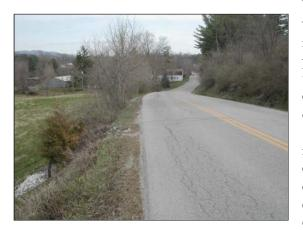
be extended. One other area of concern with regards to drainage is the stretch of road between the Putnam and DeCourval property. A steep slope immediately on the east side of the hill poses a challenging drainage situation, which will need to be engineered if the road is to be widened (show in picture at left). There are also many areas along this road that either drop-off from the pavement edge, or are ditches that carry water, which will require design and engineering for drainage conveyance.
