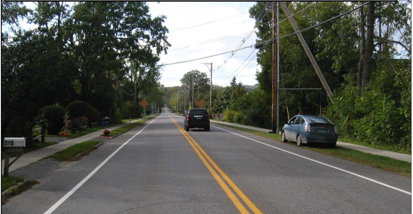
FIGURE 4: Harbor Road (SHEL-25) East of School Driveway ~ Westbound, 2012
