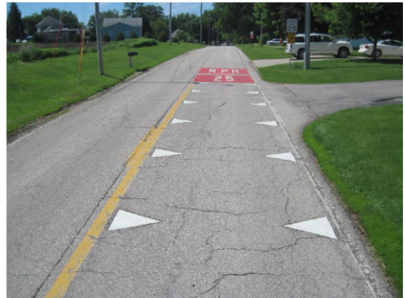
Figure 8: Optical speed bars (left) and Dragon's Teeth (right) application. (NCHRP Report 737)
