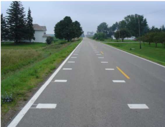
Figure 8: Optical speed bars (left) and Dragon's Teeth (right) application. (NCHRP Report 737)
