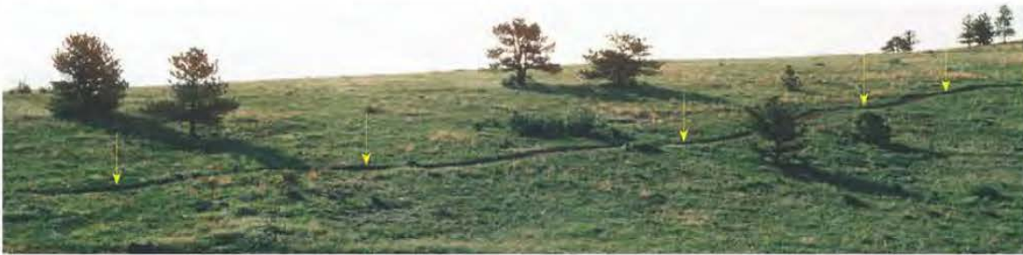
Gentle slopes require careful attention to draining tread dips. Without a steeper slope to quickly drain the dips, puddles and mudpits can quickly form.
