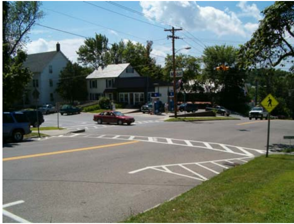
Figure 16: The Southern Corner of the Intersection
