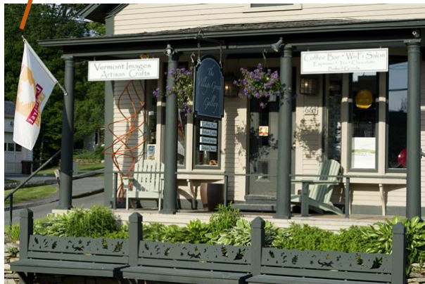
Community or commercial building
