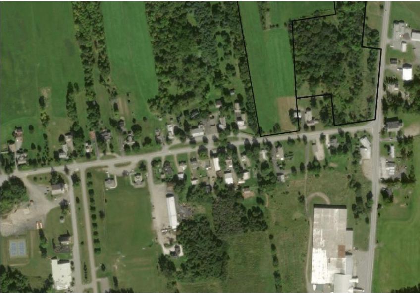
Aerial View of Shoreham Village
