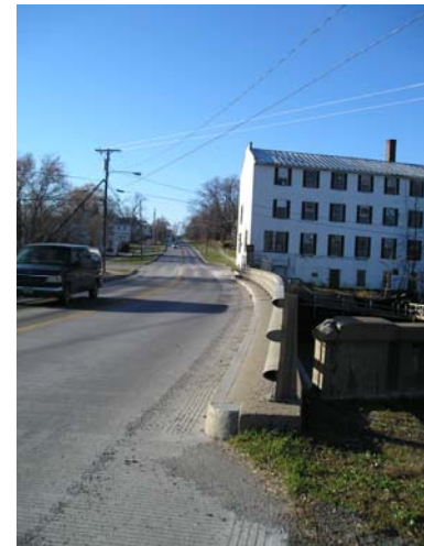
VT 22A – Looking South
