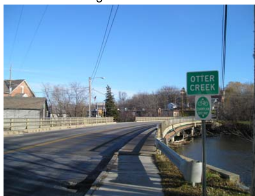
Otter Creek Falls Bridge
