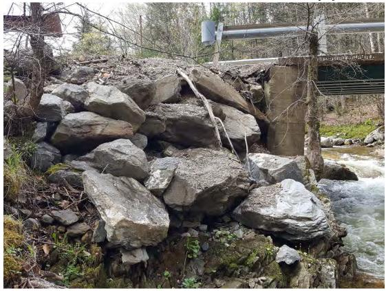
• The approach rails are not continuous with the bridge rails. The backfill at the eastern abutment consists of boulders.
