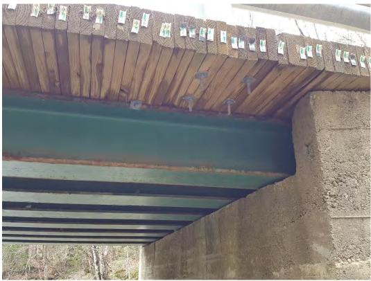
• The steel stringers and timber deck are in good condition
