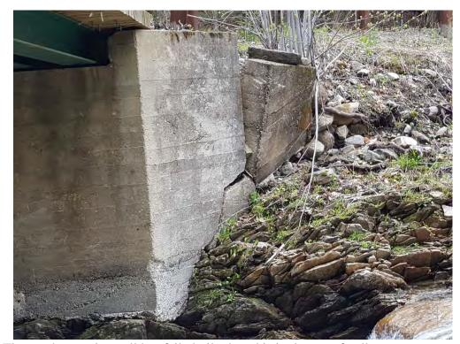
• The southeast wingwall has failed, tilted, and is in danger of collapse.
