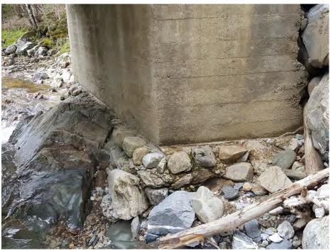
• On the western abutment, there is a "mud slab" consisting of mortar and stone between the concrete and the bedrock which interferes with contact and bond.
