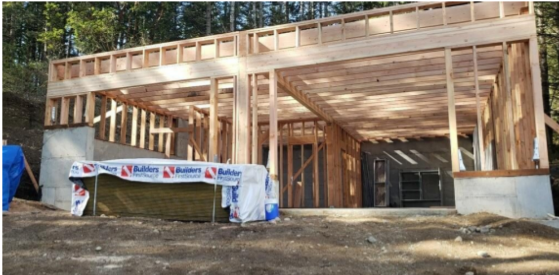
Attached new garage and ADU under construction
