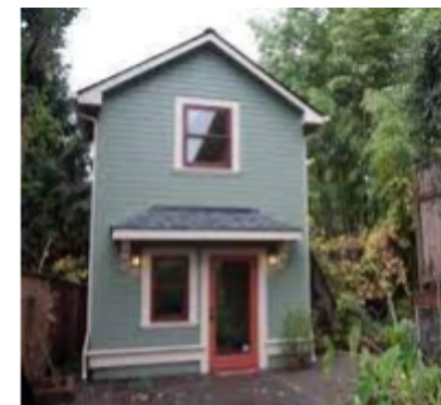
Detached new construction ADU
