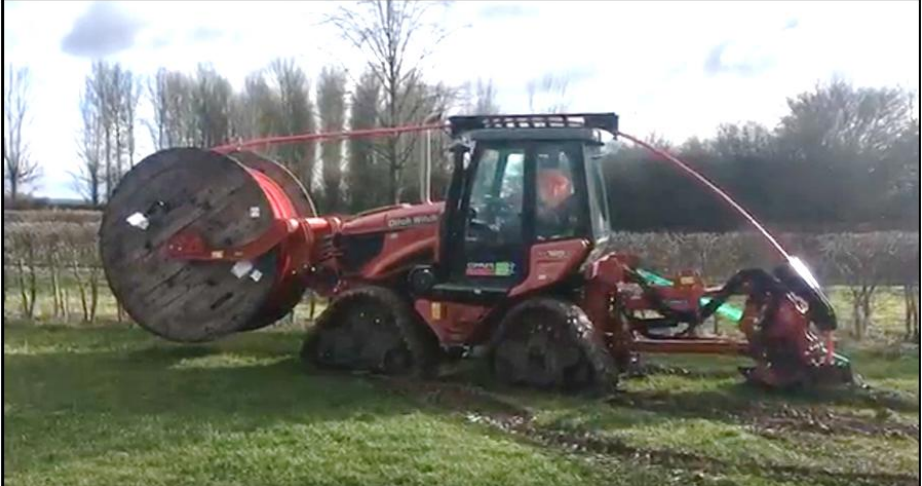
Underground installation-Vibrating Plow
