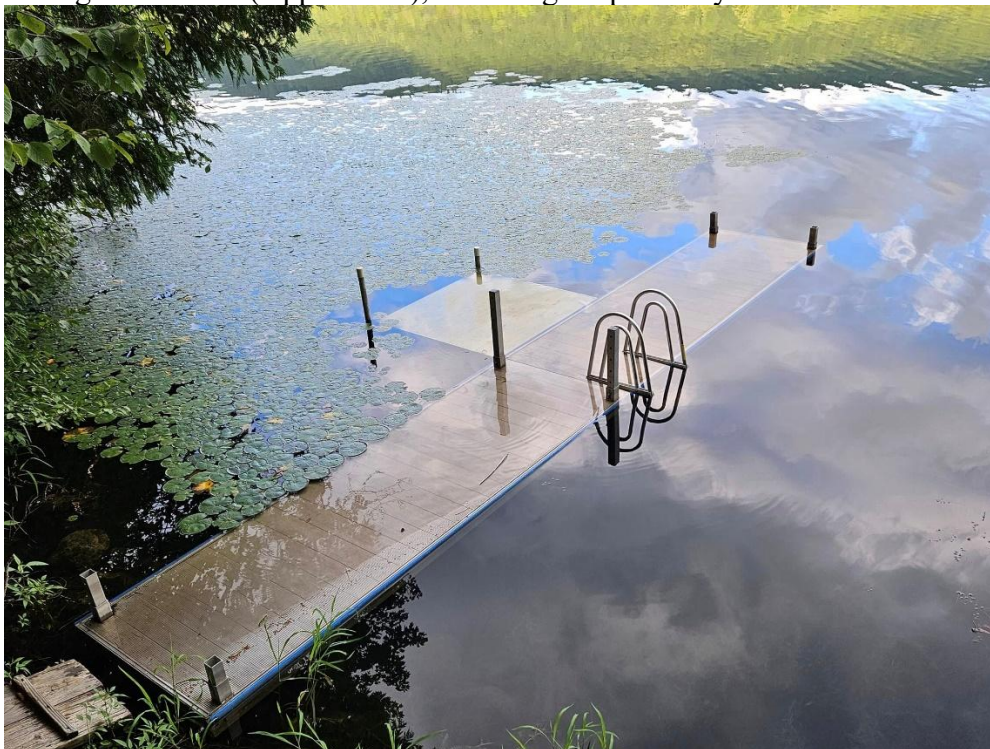
Figure 1. Dock on Fern Lake, during flooding of August 2023
