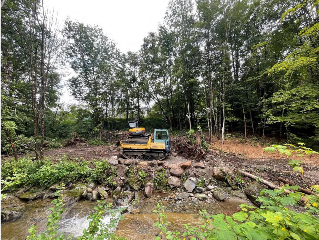
FRCF-funded old-bridge abutment removal to restore floodplain, Hollow Brook, Starksboro Vermont
