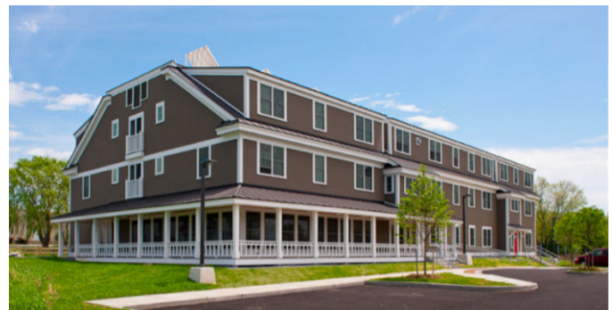
Figure 32: Armory Lane, Vergennes
