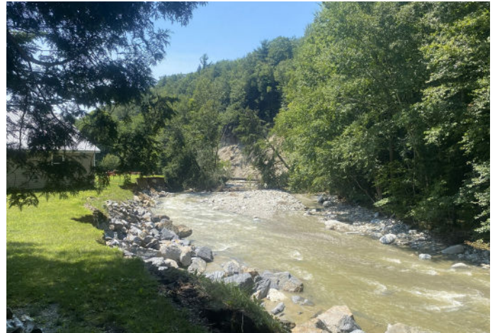
Lewis Creek erosion along Ireland Road, Bristol-Starksboro
