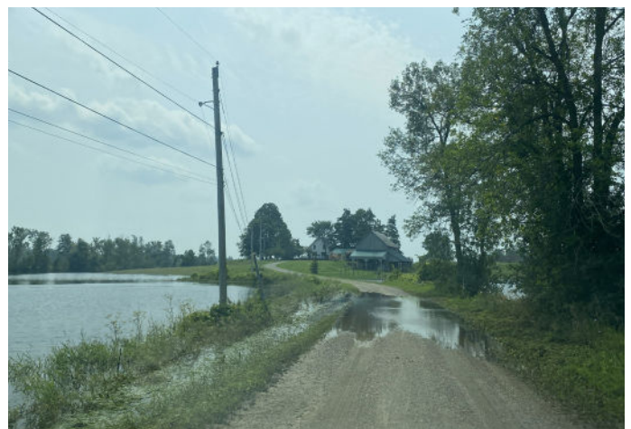
Middlebury, South Street Extension
