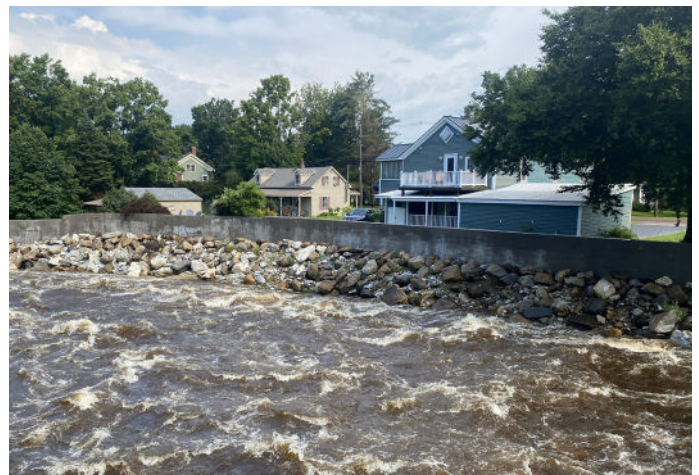
Middlebury River Flood Mitigation Project, East Middlebury
