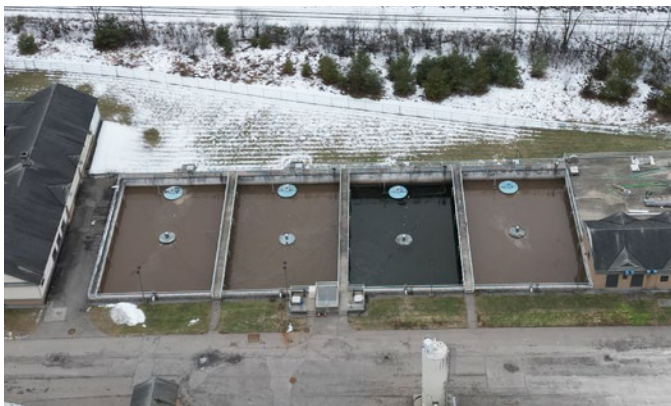
Middlebury Wastewater Plant
