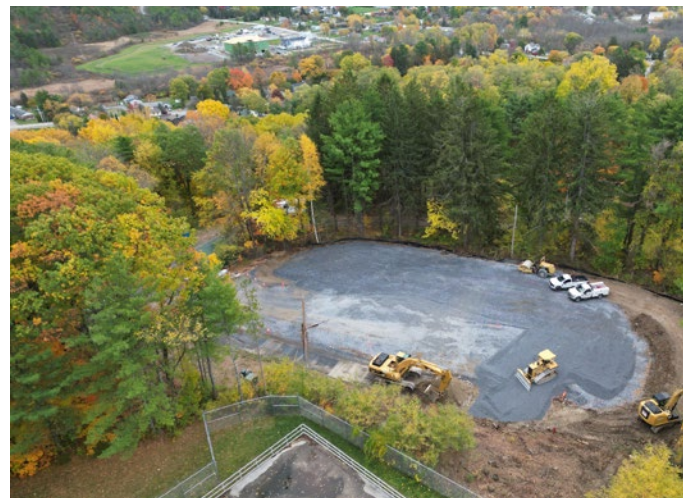
Middlebury Reservoir Construction
