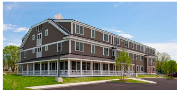
Figure 30: Armory Lane, Vergennes
