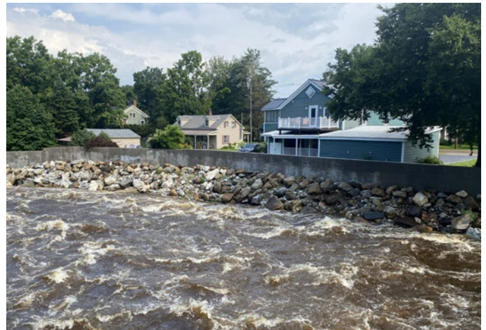
Middlebury River Flood Mitigation Project, East Middlebury
