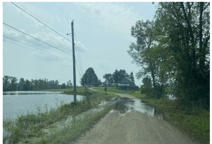
Middlebury, South Street Extension
