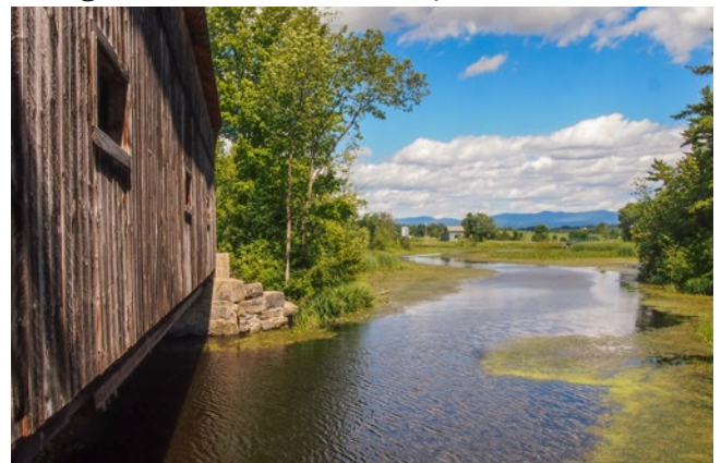
East Shoreham Railroad Covered Bridge
