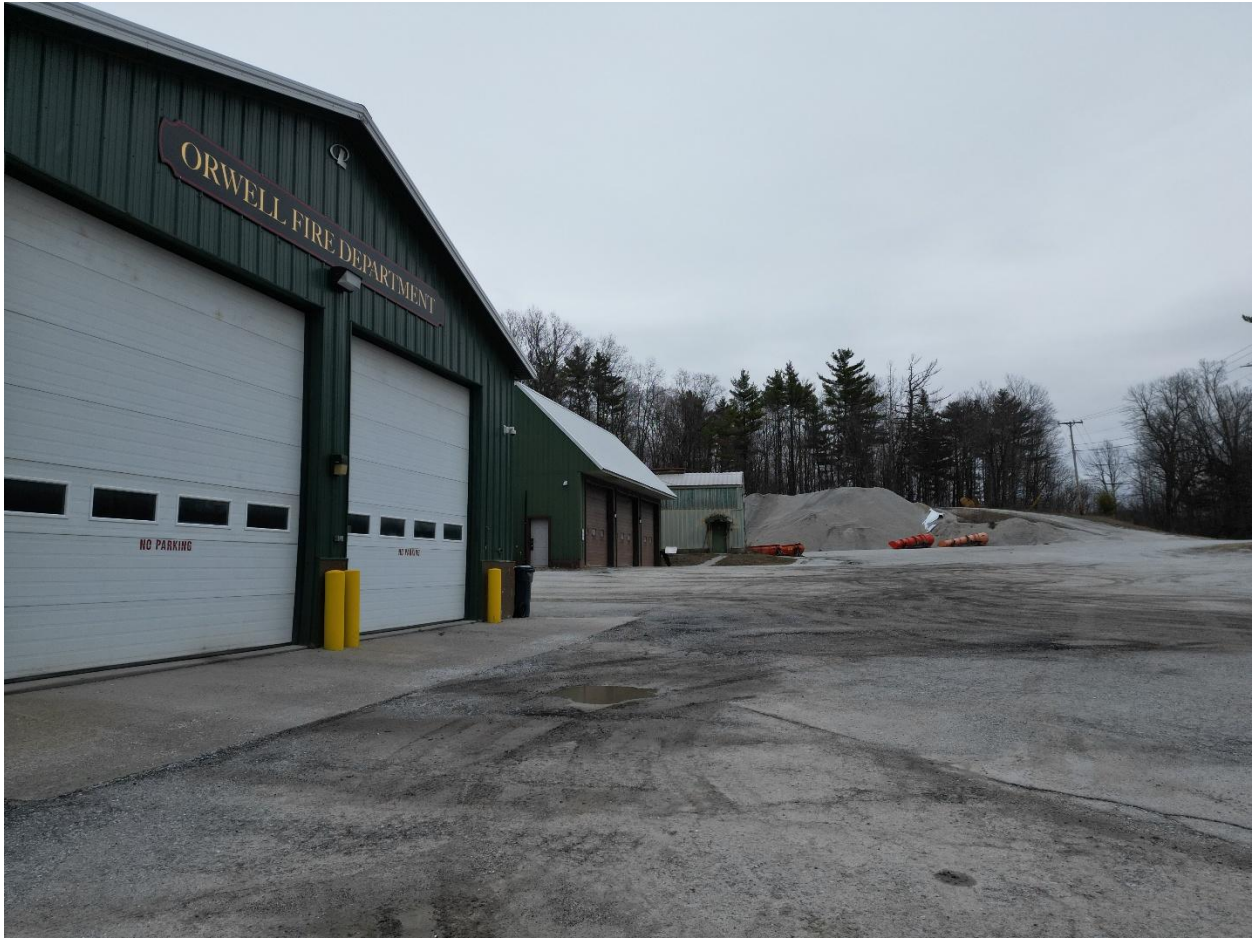
Orwell Fire Department and Town Garage
